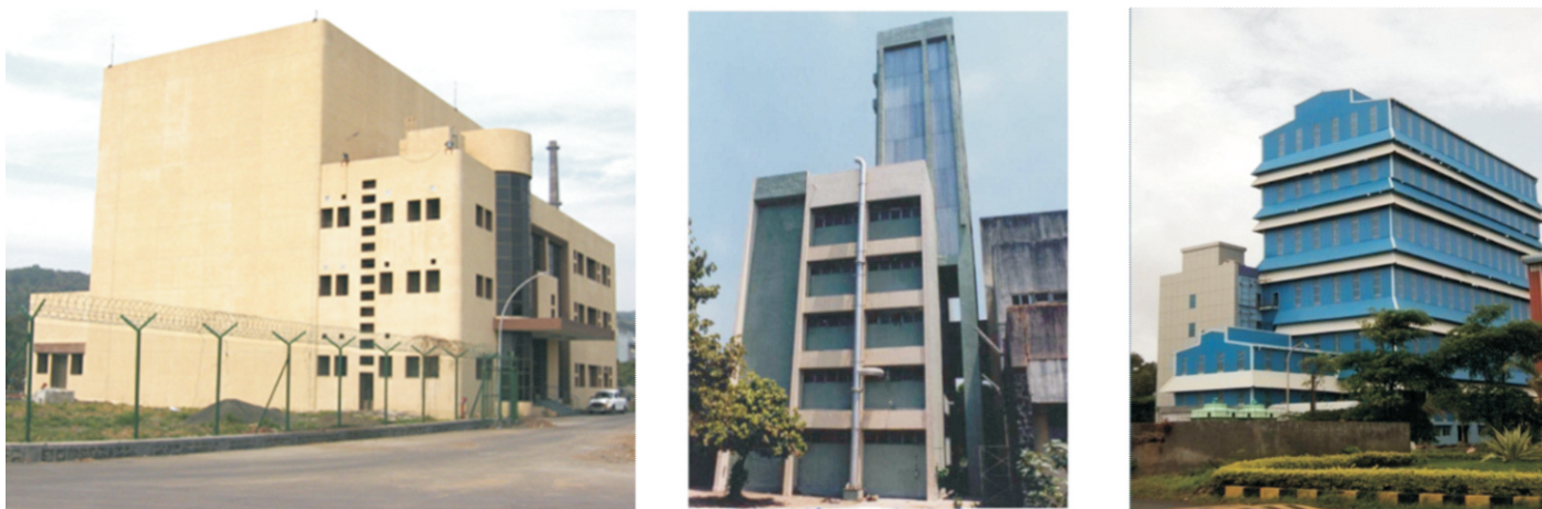
Figure 3: Installations having Critical Facility, Integral Test Loop and PARTH
